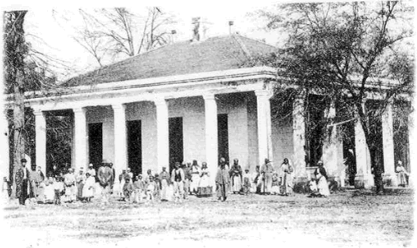
Hurricane Garden Cottage at Davis Bend. Photograph from the J. Mack Moore Collection, Old Court House Museum, Vicksburg, MS, which cannot be reproduced without consent.
